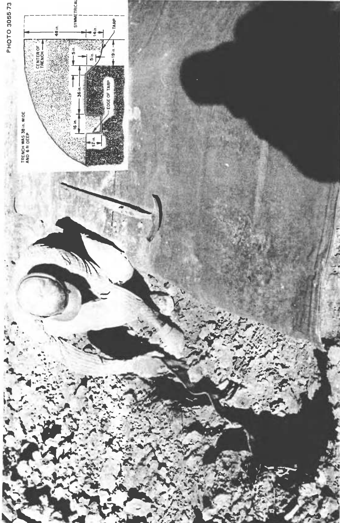
Fig. 3.11. Building the best of two successful Tarp-Roofed Trench Shelters constructed on Dec. 1, 1973, on the Kearny farm near Montrose, Colorado. C. H. Kearny designed this shelter after the November tests of the Door-Covered Trench Shelter had convinced him that, if the principles of earth arching and friction are used properly, then blast shelters can be built in many areas by roofing a trench with only a tarp or a strong rug, and then intelligently covering the tarp or rug with earth.
