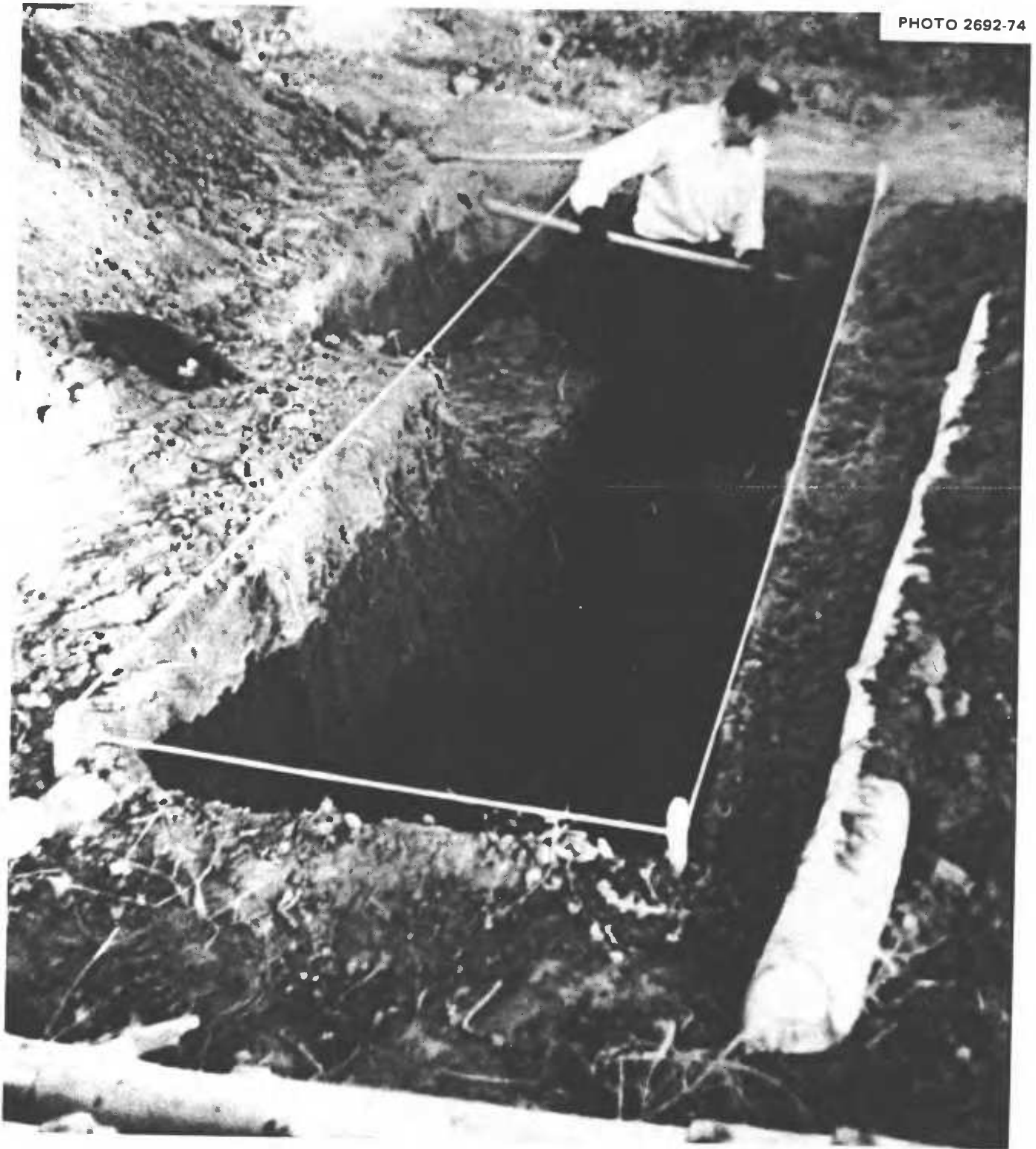
Fig. 4.4. Expanding the shelter room to its full specified width of 3\frac{1}{2} feet, and to its 4\frac{1}{2} -ft depth. This intelligent man made unnecessary work for himself by not following the instructions to cut a 3\frac{1}{2} -ft stick, and then use it repeatedly to be sure the trench was being dug full width.
