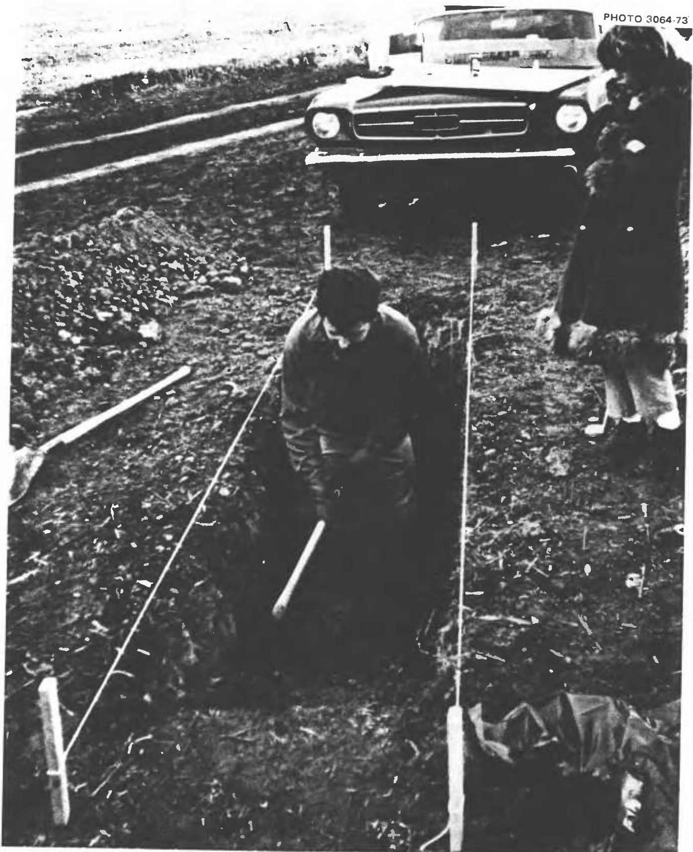
Fig. 6.6. The father swung his pick properly, a result of his learning to use an ax as a boy of 12, when his family spent a while in rural Oregon. However, he tied unnecessary strings between the stakes, and left them tied, and dug the trench too narrow. Later, he spent about two hours inefficiently widening it.
