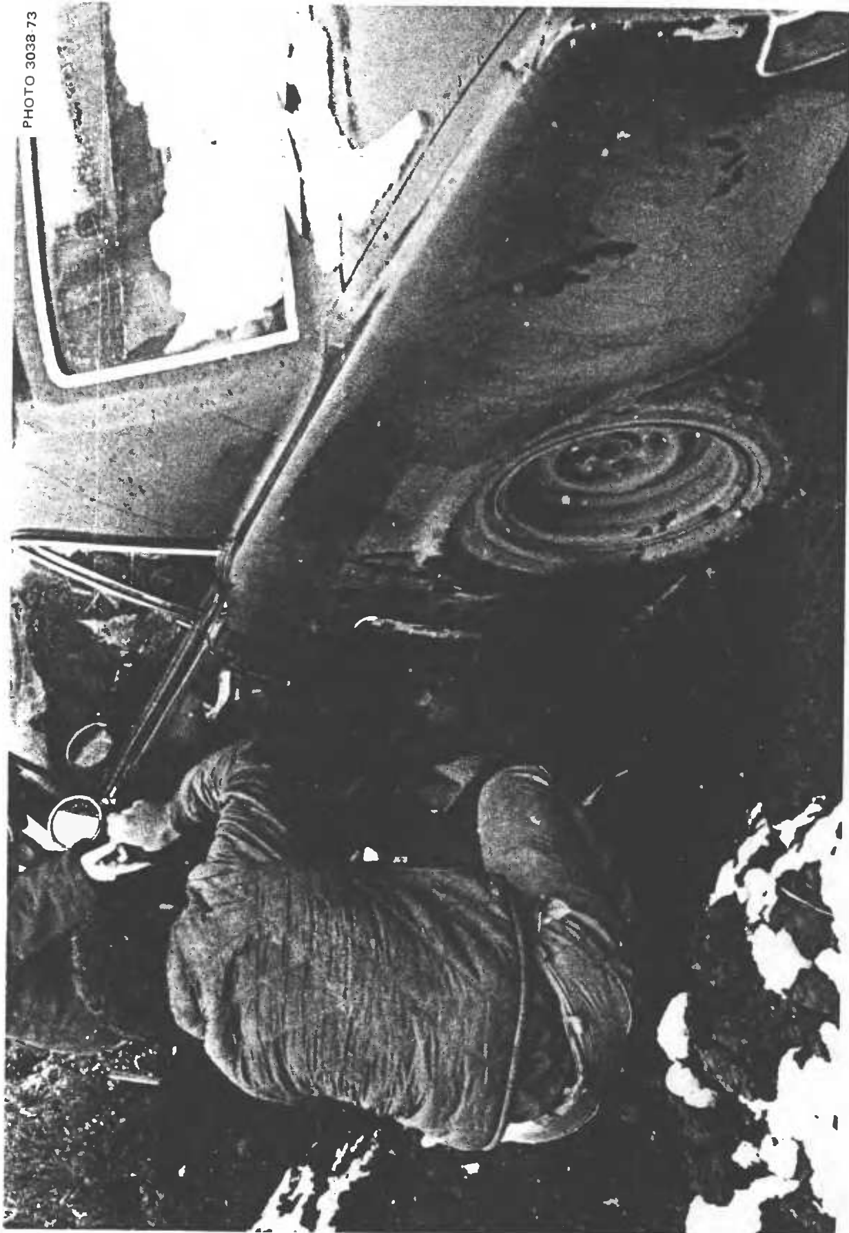
Fig. 6.12. Taping split-open plastic garbage bags to the sides of the car, for want of other waterproof material to keep some of the dry earth to be mounded around the car from running under the car onto the storage "shelf" areas around the edges of the trench, or into the trench. Fortunately, the father had some waterproof duct tape, and cleaned the dirt off the spots on the car to which he planned to tape the plastic. However, because he did not tape all of the upper edges of the pieces of plastic, if water had run down the sides of the car, much of it would have run under the upper edges of the plastic and into the shelter space under the car.
