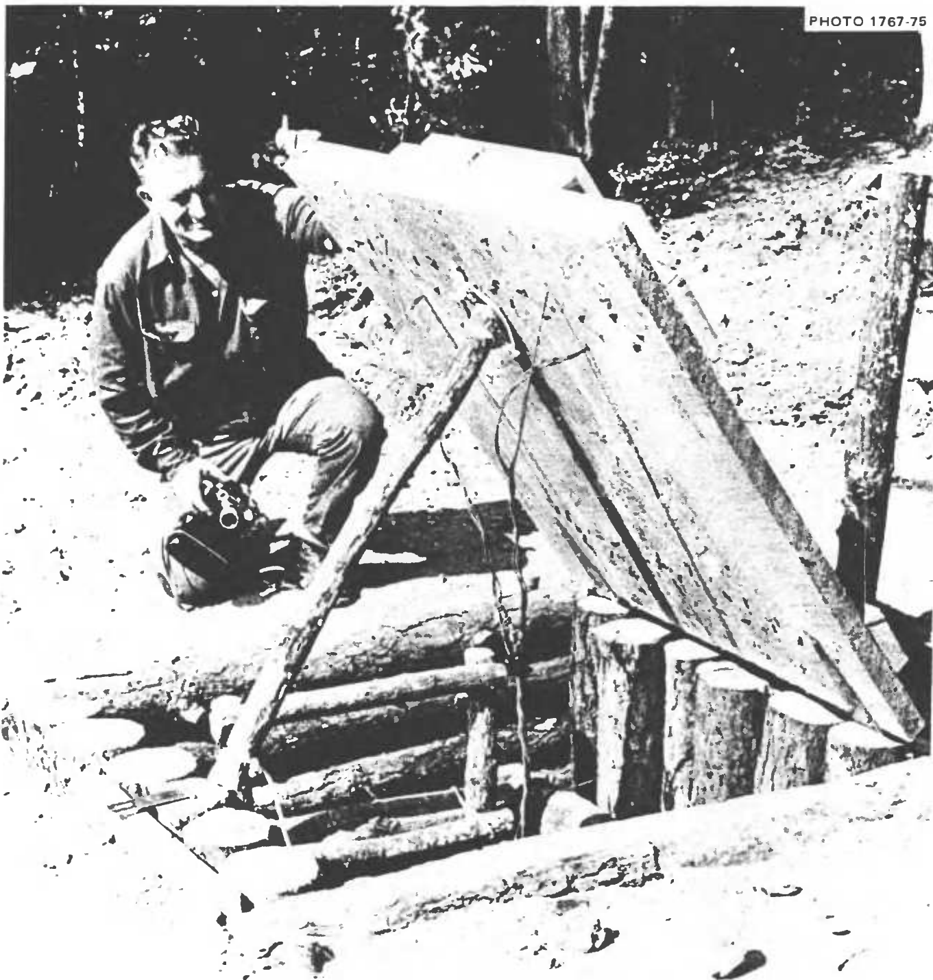
Fig. 7.4. One of the two completed vertical entries, with its expedient blast door made of 2-in.-thick rough lumber. Its hinges were made of strips of worn auto tires, spiked to each of the vertical entryway posts on the hinged side. A door of this type successfully withstood a blast overpressure of 17 psi.* The other blast door was made of 3-in. planks and may have been able to withstand higher blast over pressures than would collapse the earth walls of this covered-trench shelter.
