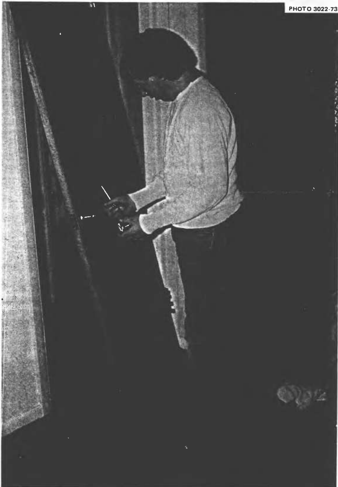
Fig. 2.1. Start by an untrained, unskilled family of the second proof-testing of the written instructions for building a Door-Covered Trench Shelter. Starting at 6 AM on November 24, 1973, son Tad, age 14, and other children removed the doorknobs from one of the six interior doors that this fatherless family of six readied for use.
