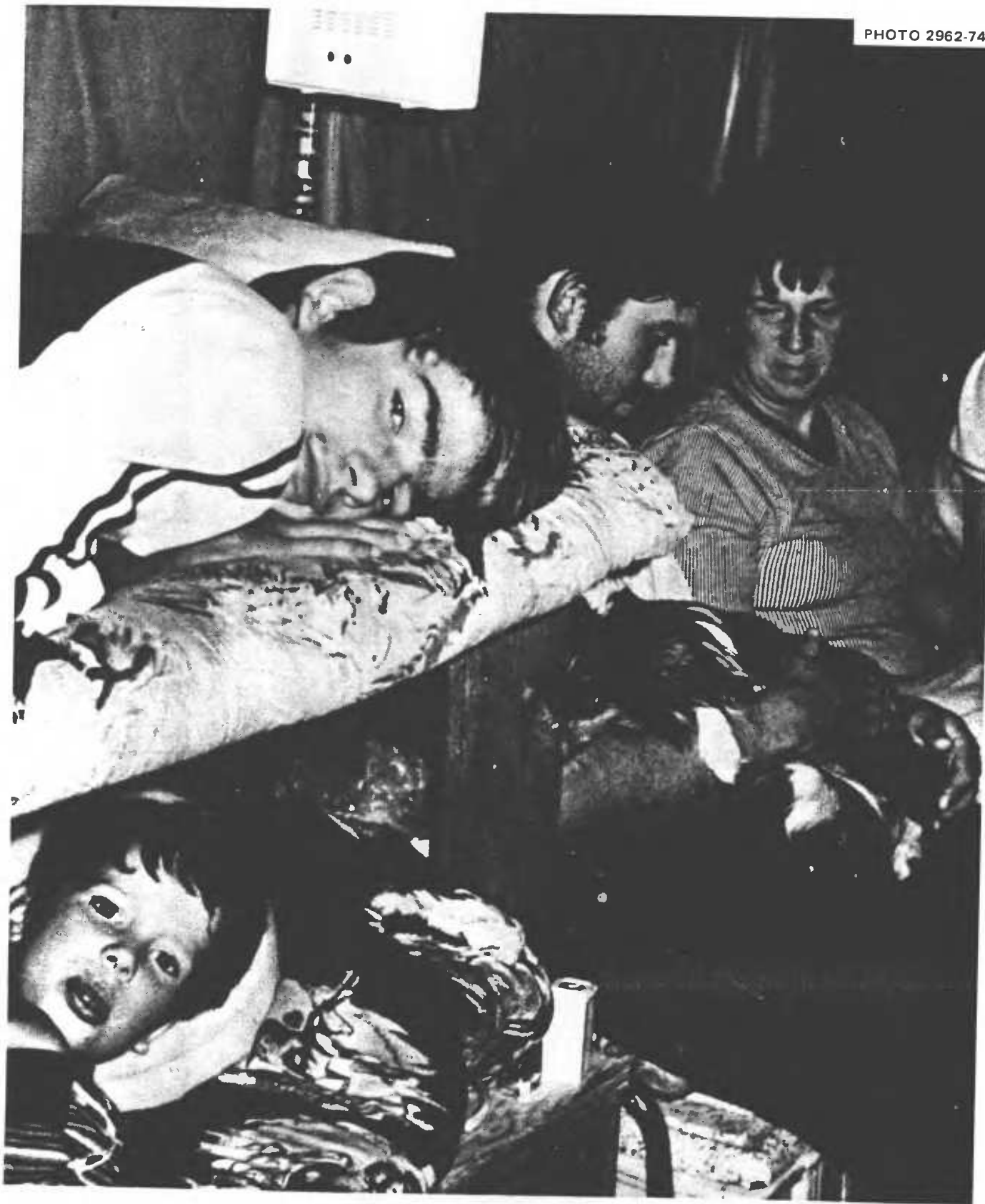
Fig. 4.12. Inside the completed shelter, showing the double-deck bunk, 21 in. wide and 6 ft long, in the 42-in.-wide shelter room. Most of the time two of the six shelter occupants slept or rested on the two bunks, while the remaining four sat in the four chairs along one wall. The walls were covered with 1-mil polyethylene sheets cut from garbage bags. This plastic was also placed under the shag rug on the floor, to keep the damp earth from dampening the rug.
