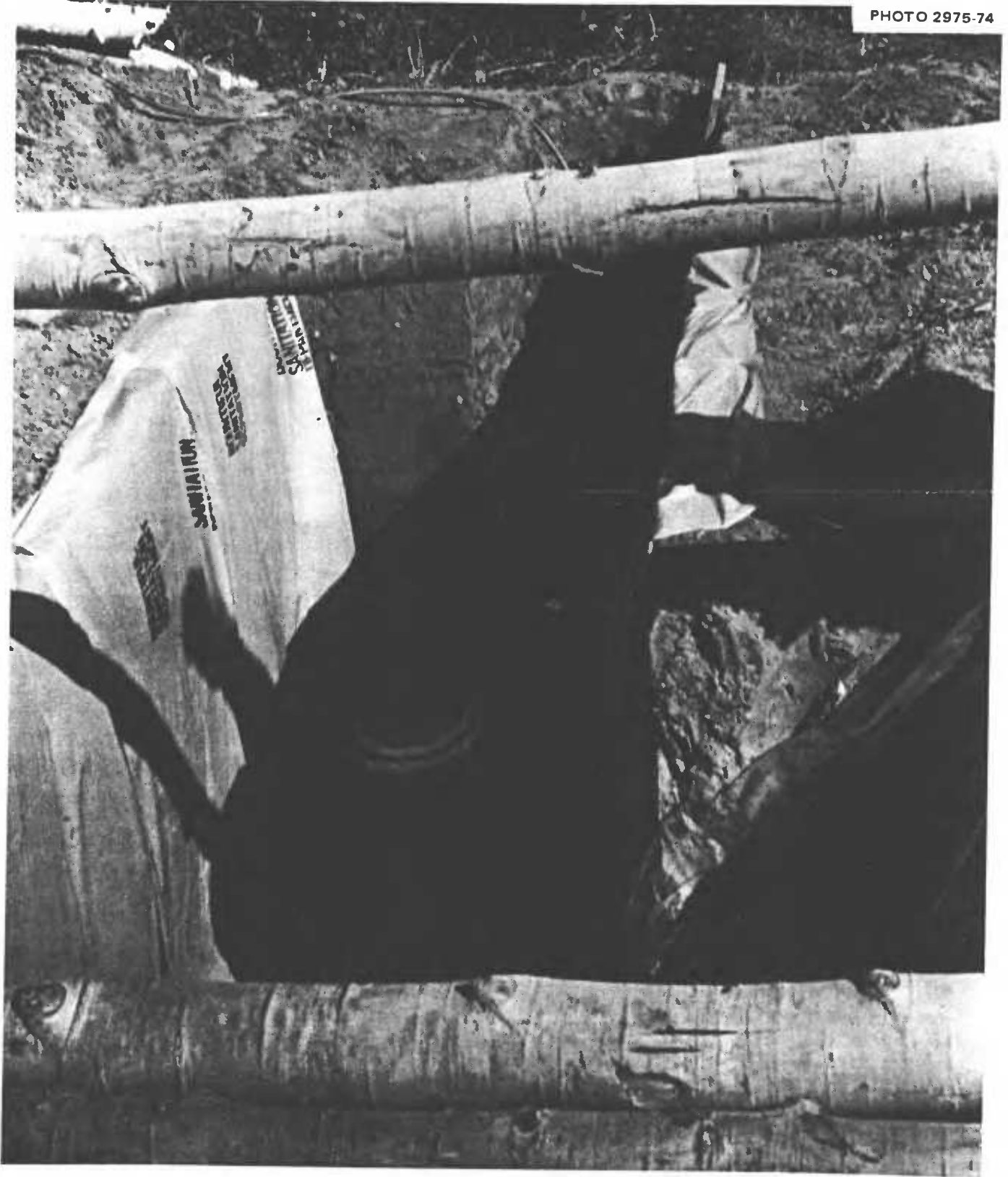
Fig. 4.6. Covering the main trench with 9-ft aspen logs. These logs were 4 to 6 in. in diameter at their small ends – thus being stronger than necessary to support the planned 3 ft of earth cover.
