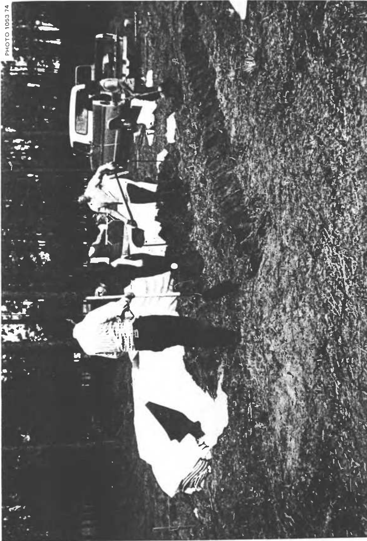
Fig. 5.4. Starting to make the first roll by shoveling earth onto bed sheets that had been placed with 2 ft of their long sides on the ground, with the rest of the sheets temporarily draped over the doors used as forms. This sandy earth could be dug quite easily with shovels.
