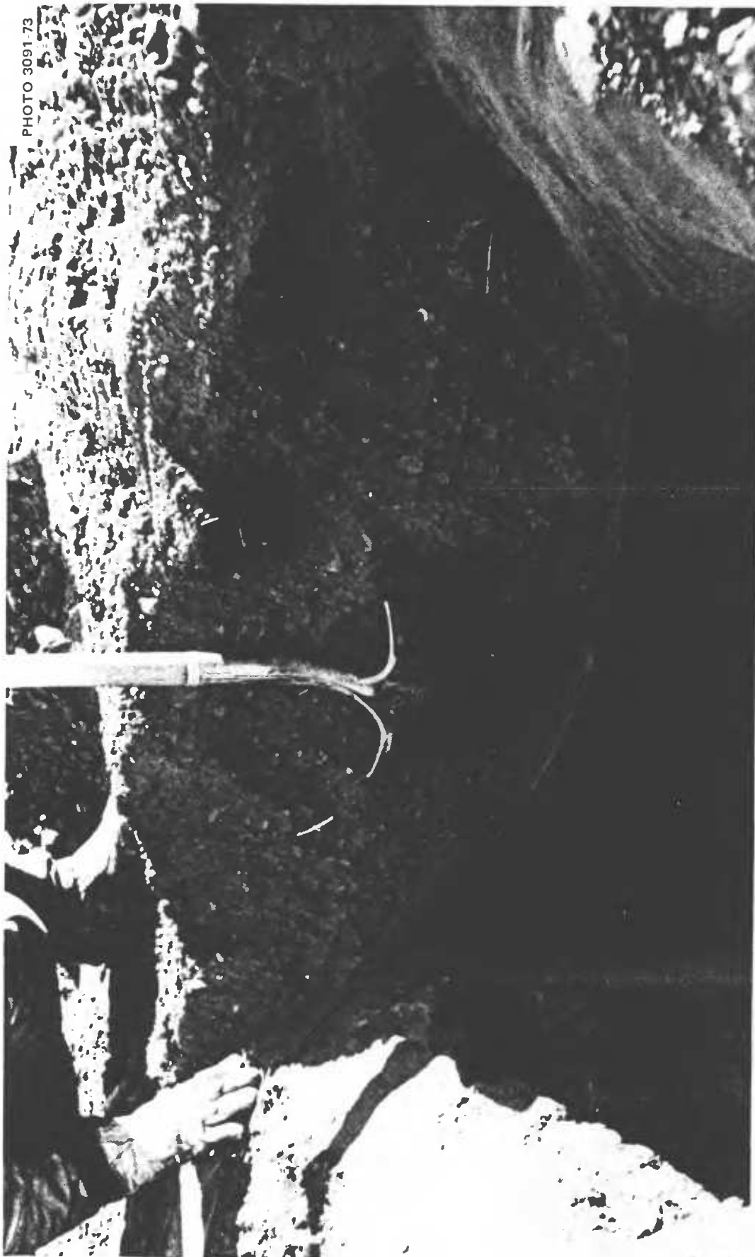
Fig. 3.15. View of the tarp catenary after the backhoe (that was removing the earth cover) had accidentally snagged part of the tarp and torn it. Note the 45° beveled edge of the trench.
