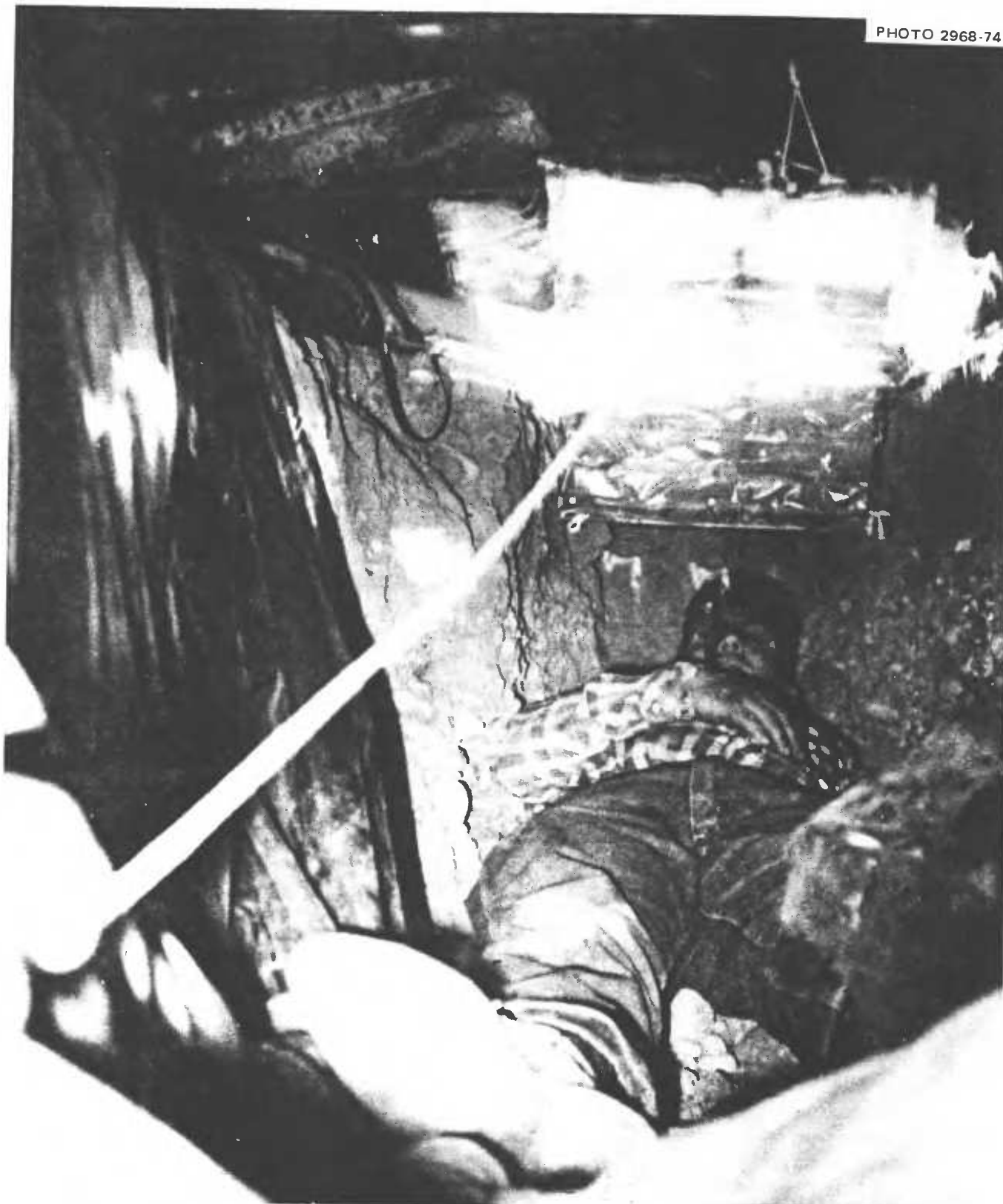
Fig. 6.16. A 17 X 19 in. KAP being used to pump about 100 cubic feet per minute through a Car-Over-Trench Shelter, and out through the 110 square inch exhaust opening. Especially during hot, sunny weather, temperatures inside a Car-Over-Trench Shelter would become intolerable without adequate forced ventilation.
