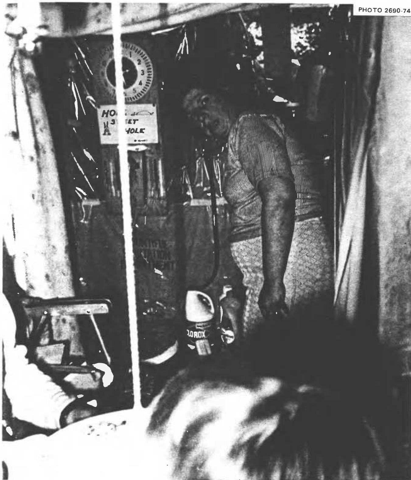
Fig. 4.23. The mother standing in the 18-in.-deep stand-up hole next to the toilet. Note the air-duct-emergency exit, shown above the mother's shoulders, with a piece of toilet paper hanging from its roof to indicate air movement.
