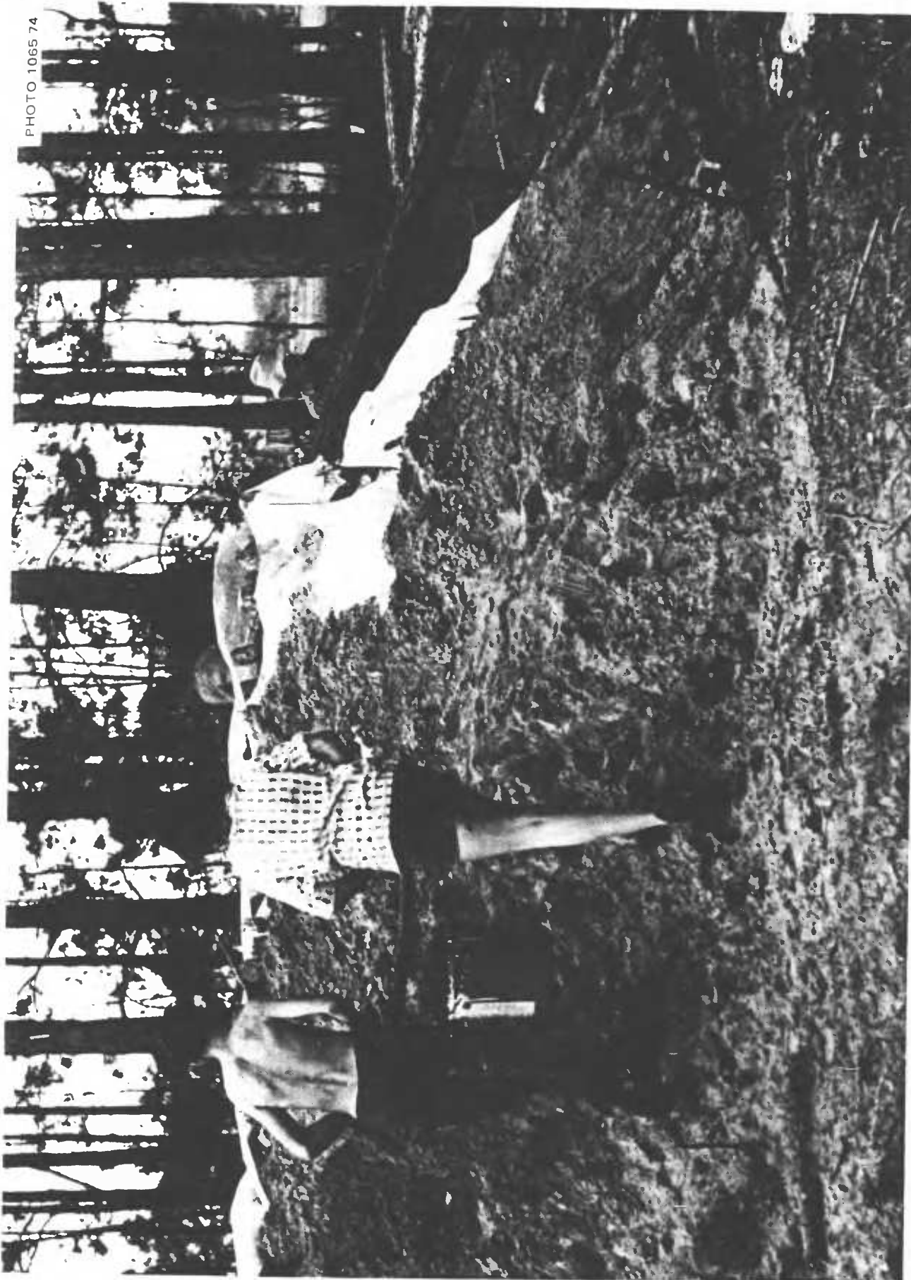
Fig. 5.36. Two teenagers carrying earth in a 5-gallon bucket, from one of the shallow barrow pits. These builders found that carrying earth in this manner enabled even children to move earth effectively, all the way to the top of the shelter.
