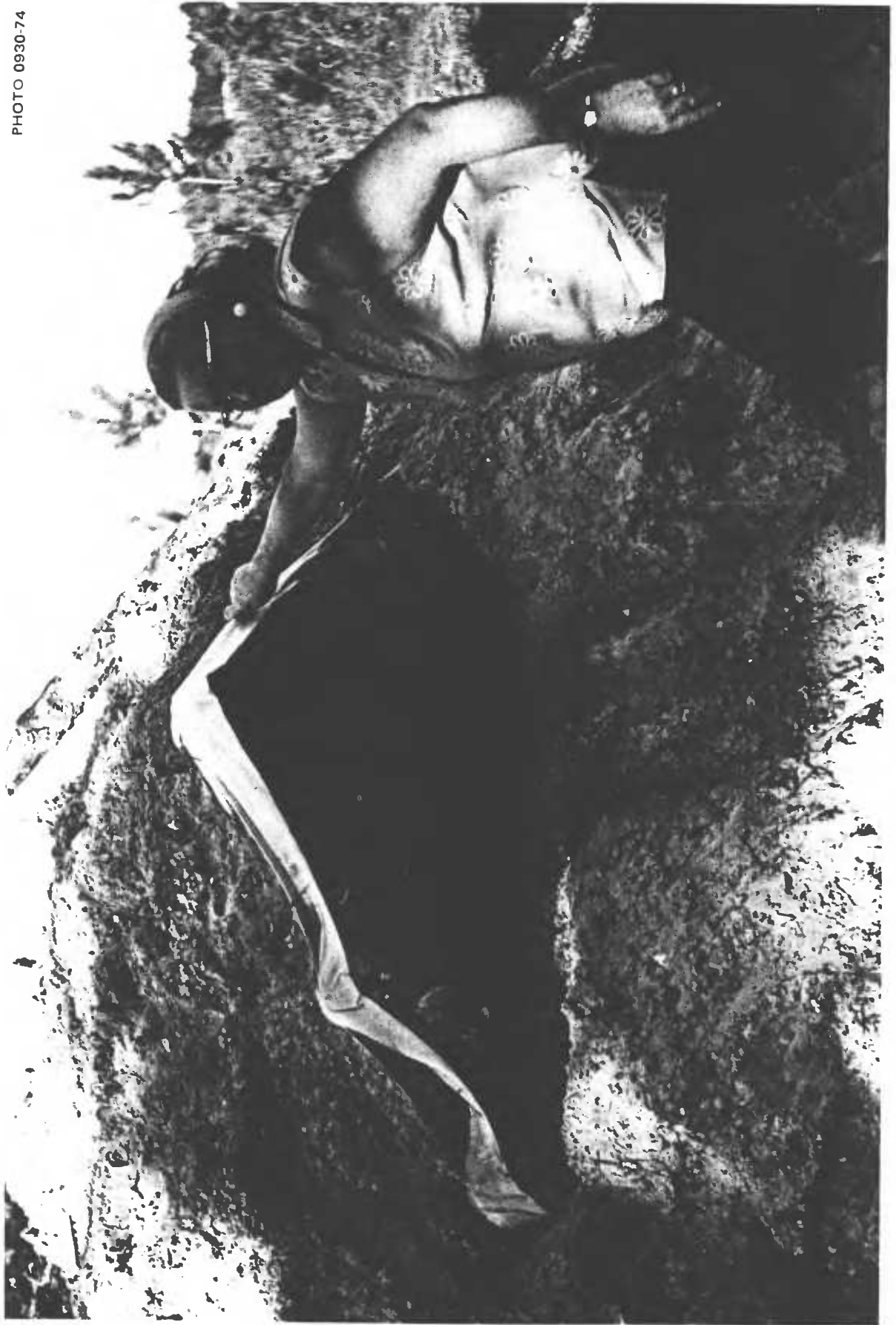
Fig. 5-50. The simplified, but not as protective, ventilation opening constructed in what had been the end of the shelter toward which the skewing movement occurred. Seven-foot poles were placed on the roof poles, parallel to the ridge board and extending 3 ft beyond the outermost wall poles. Those 7-ft poles formed the overhanging gable shown in this photo. Later, the earth cover was thickened.
