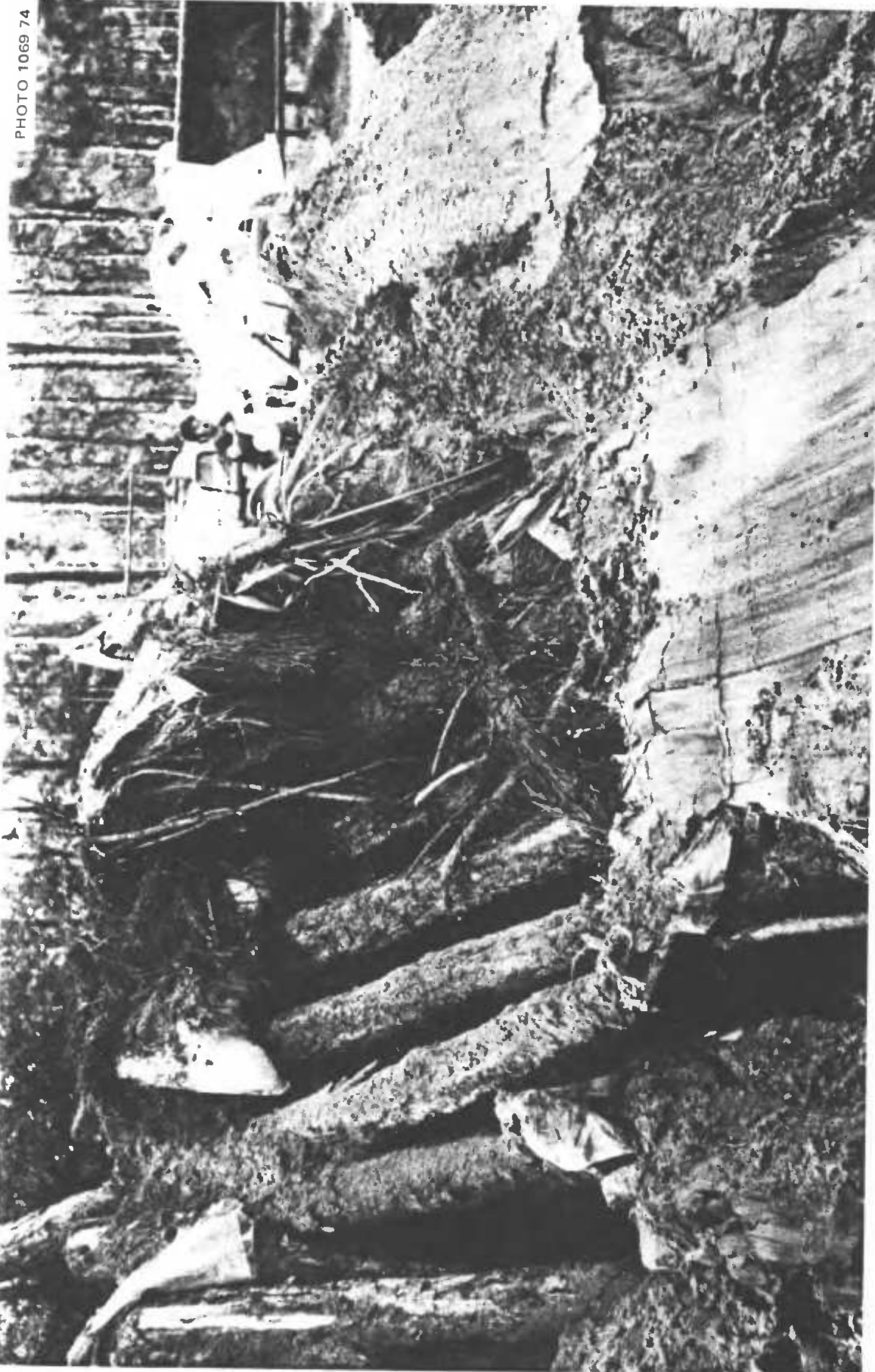
Fig. 5.40. View after a backhoe had started to demolish the Waldens' Ridge-Pole Shelter, which proved to be decidedly sturdy. Note that some of the wall poles were broken before they were moved off the ridge poles, or the ridge pole had been moved significantly.
