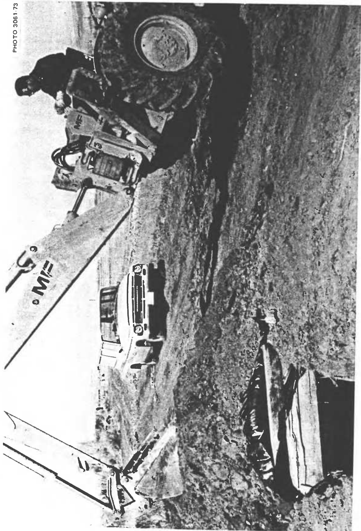
Fig. 3.13. Stressing the Tarp-Roofed Trench Shelter, a 6-ton backhoe, supported only by its buckets, pressed down repeatedly with its front bucket on a 62-in.-deep mound of loose earth. The mounding of loose earth caused the tarp to bow downward (sag) into a catenary curve. The compaction caused the tarp to stretch, resulting in an increase of the maximum sag from 8 to 14 in.
