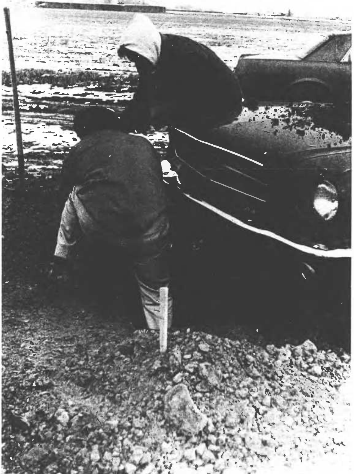
Fig. 6.13. Placing earth-filled plastic garbage bags around the edges of the entryway trench. The mother was able to remain on the site all of the second day and do some work – thanks to a borrowed pair of insulated boots that kept her feet from getting painfully cold.
