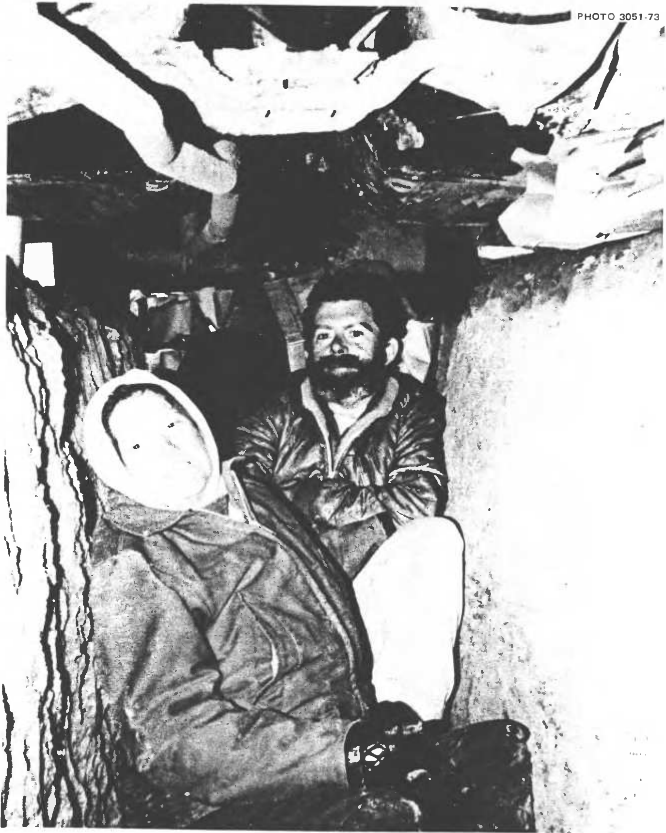
Fig. 6.15. The father (sitting on a box) and the mother in their 40-in.-deep, 28-in.-wide shelter. Enough room remained (occupied by the photographer's leg when this picture was taken) for the small daughter and the family poodle. All of their supplies had been placed under the car.
