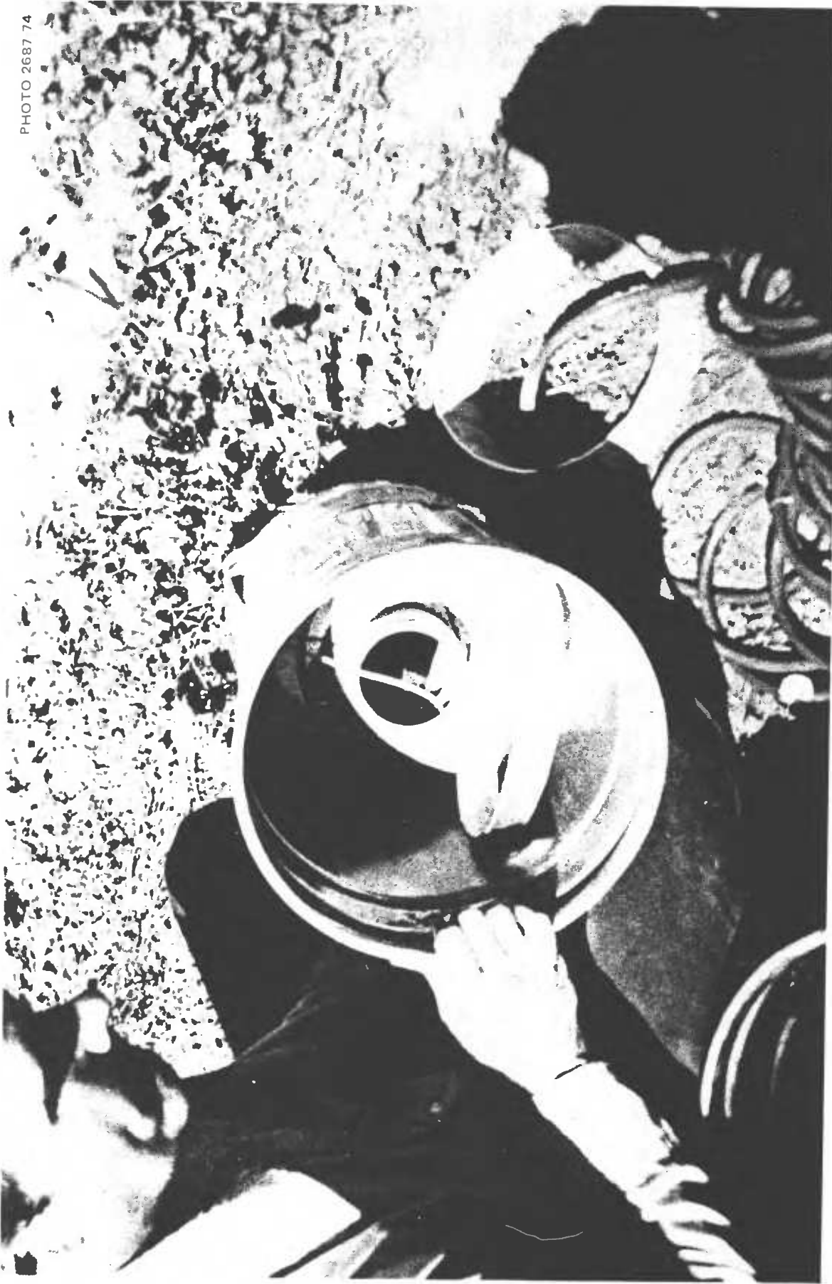
Fig. 4-27. View looking into what was to become the uppermost 5-gallon can of the 10-gallon vented space. The toilet bowl is on the ground, below this can and attached to it. The mouth of the shortened, plastic water-jug bowl is shown extending through the hole cut into the bottom of this can. Freezer tape had been used to seal the cracks between these parts.
